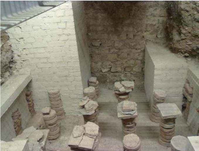
View of the tile pillars, which stand on the sub-floor at regular intervals. The upper end of the pillar is formed by several square stone slabs that increase in size, and on which the heated floor rests.
